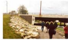
Existing grade-separated crossing at Vermillion Falls Park under Highway 61
